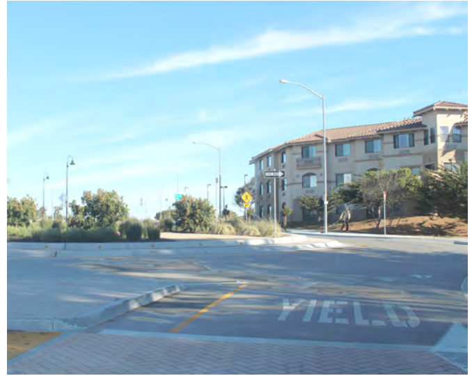
Traffic circle on Reservation Road in Marina, CA A traffic circle can provide a sense of entry. Drivers slow and plantings and civic art located within the center becomes a focal point.
