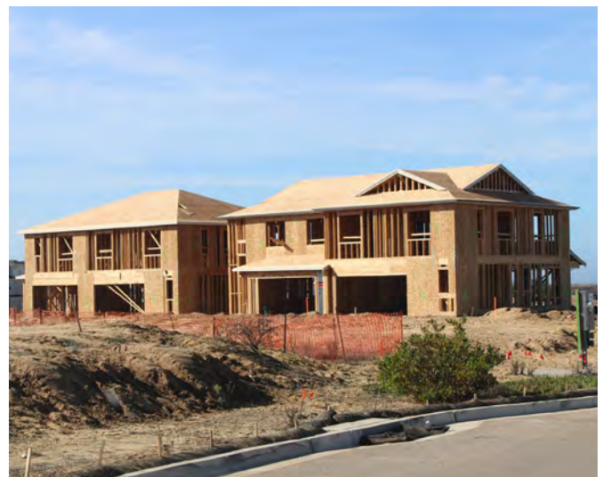
Housing Construction (Dunes at Monterey Bay)
