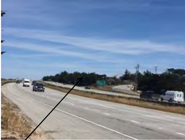
View from Highway 1 looking north
