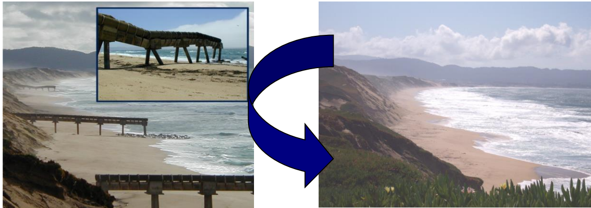
Storm drainage outfall removal – Before and After
