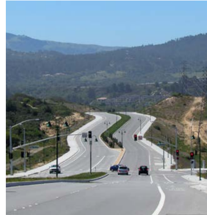
General Jim Moore Boulevard at Hilby Avenue; one of three intersections upgraded/opened in the City of Seaside
