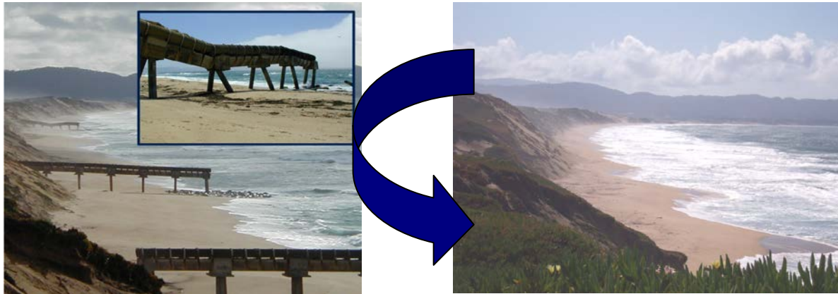
Storm drainage outfall removal – Before and After
