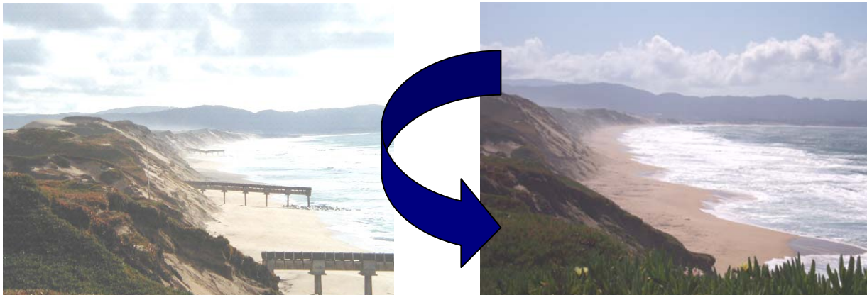
Storm drainage outfall removal – Before and After
