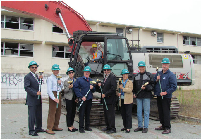
Seaside's 2018 Surplus II demolition Kick-Off event.
