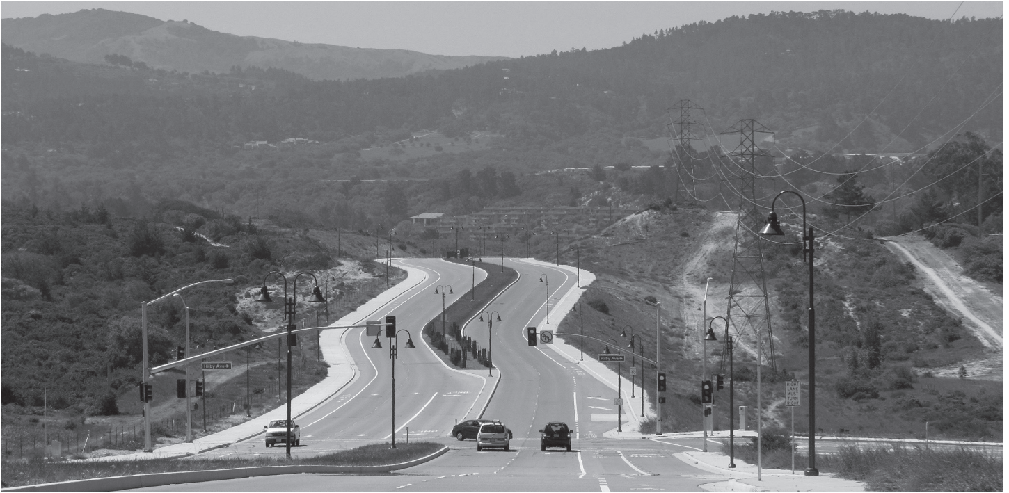
General Jim Moore Boulevard looking south from Seaside to Del Rey Oaks.
