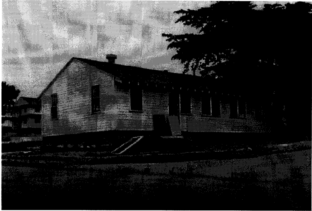
Building 1801 being prepared for relocation
