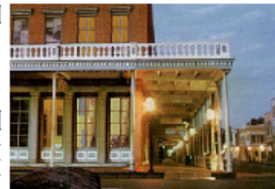
A gallery with slender metal columns.
