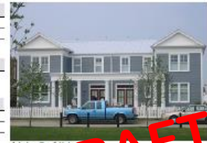
A duplex with a shared entrance.
