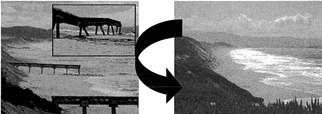
Storm drainage outfall removal – Before and After
