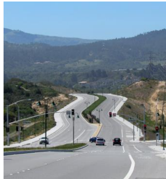
General Jim Moore Boulevard at Hilby Avenue; one of three intersections upgraded/opened in the City of Seaside
